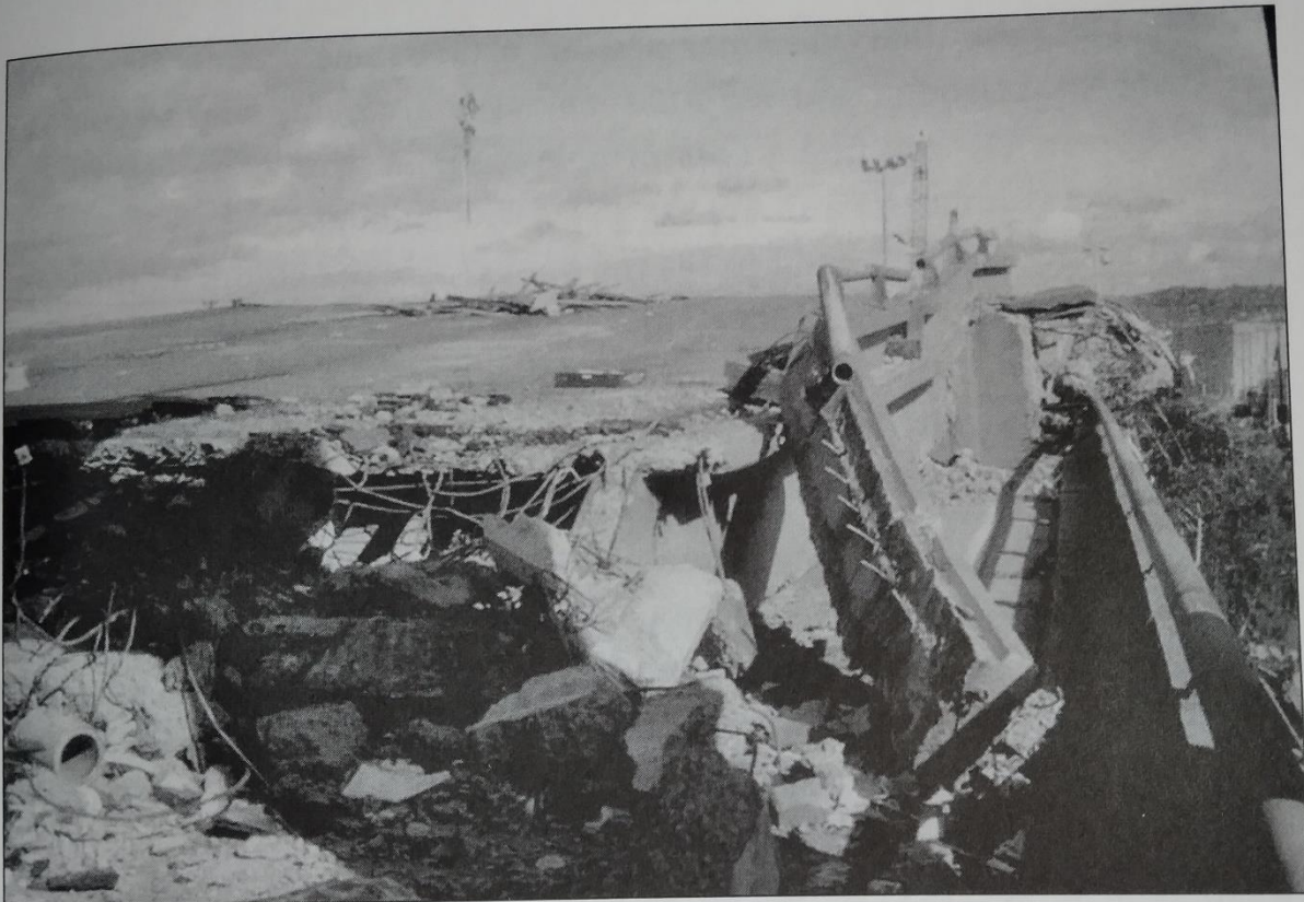
Figure 2-3. The visual message in this photo of the Cypress Viaduct in Oakland, California, after the 1989 Loma Prieta earthquake carries home the destructiveness of a powerful earthquake in ways no words can convey. (Photograph by H. G. Wilshire, U.S. Geological Survey.)
